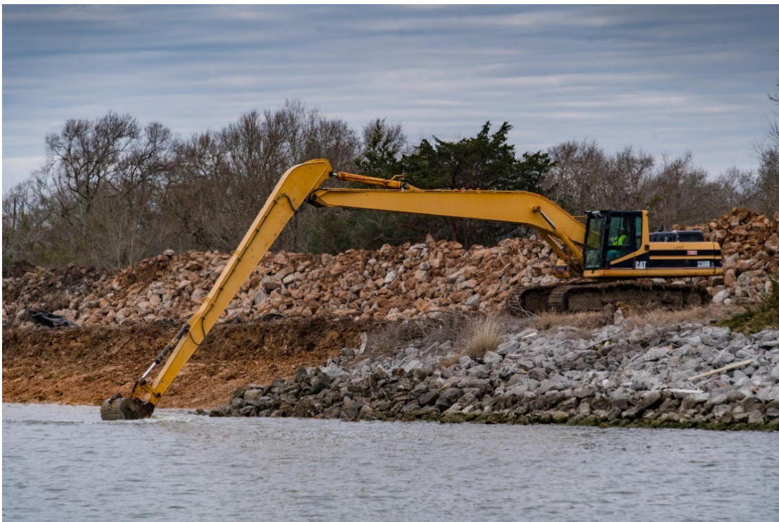
Photograph 2. Existing stone removal and stockpile
