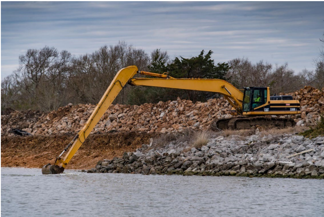
Photograph 2. Existing stone removal and stockpile
